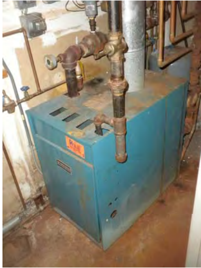
The natural gas-fired hot water boiler serving both buildings
