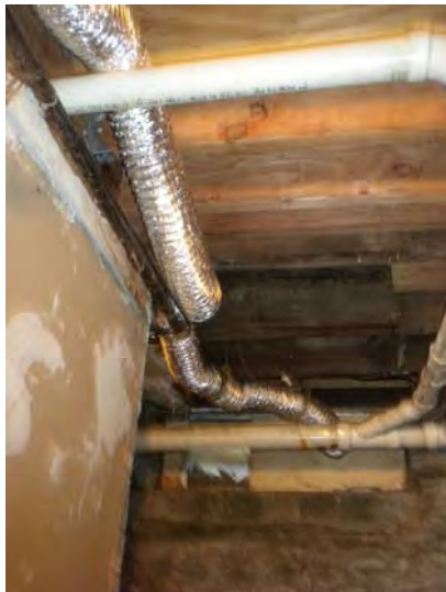
Some dryers are not properly vented
