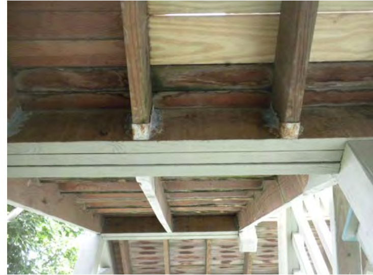
Example of framing and decking replacement at the rear fire escape
