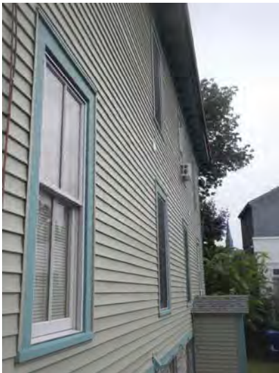
View of the new vinyl siding and windows
