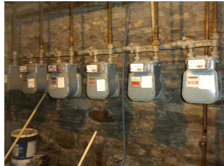
Separate gas meters for unit ranges only
